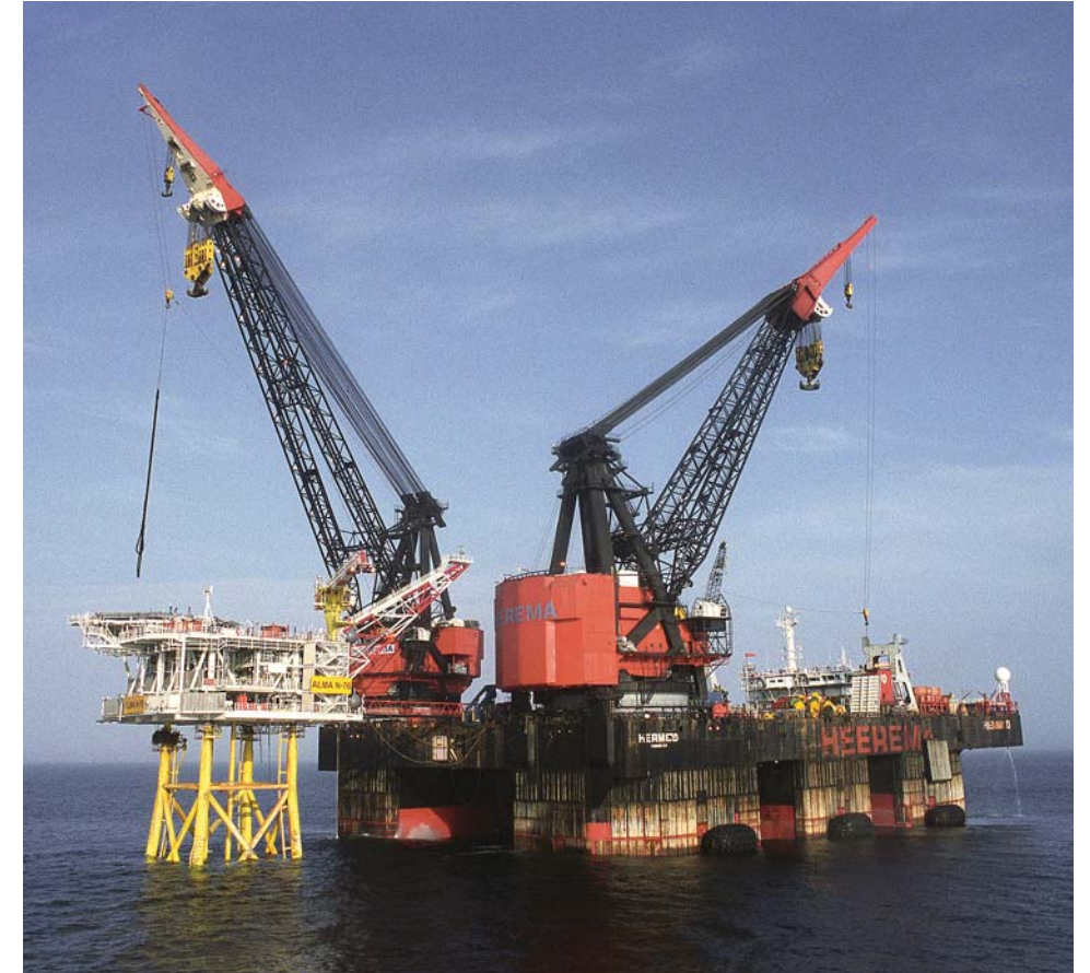
The Alma platform was put in place last summer by the heavy lift vessel Hermod.
