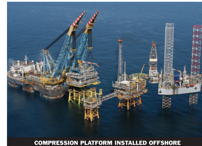
COMPRESSION PLATFORM INSTALLED OFFSHORE
